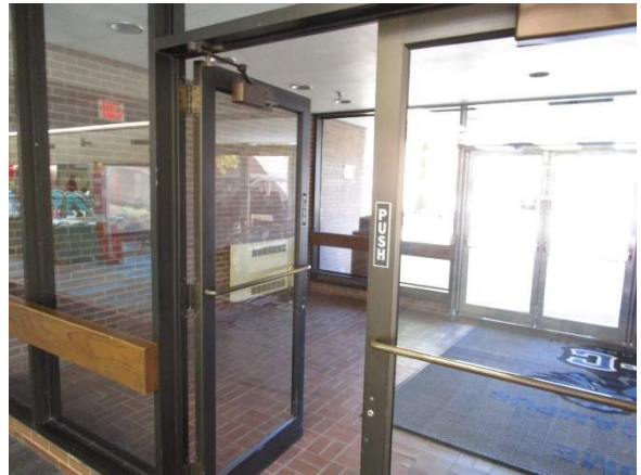
Typical Interior Aluminum Framed Doors
