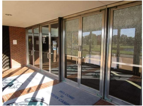
Main Theater Entrance - Interior Vestibule Doors
