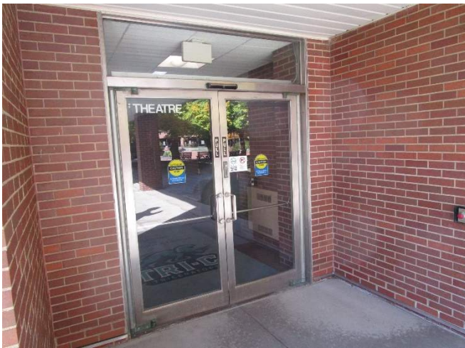
Exterior Door with Transom near room T109
