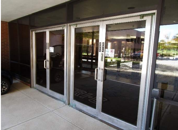
Typical Exterior Stainless Steel Doors
