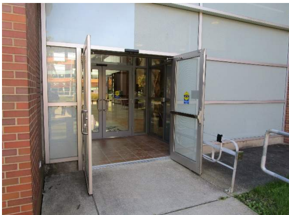
Northwest Exterior Doors to Library
