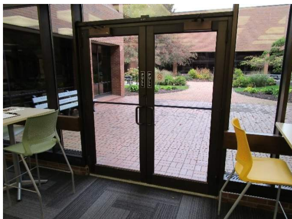
North Courtyard Doors
