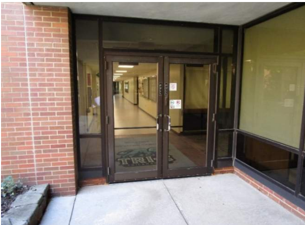
Exterior Door C100B West
