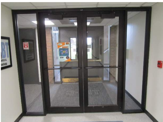
Interior Vestibule Door C100B East
