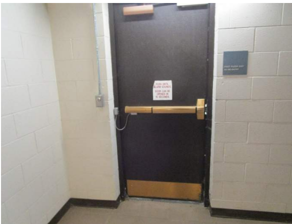
Emergency Exit Door GT111 North
