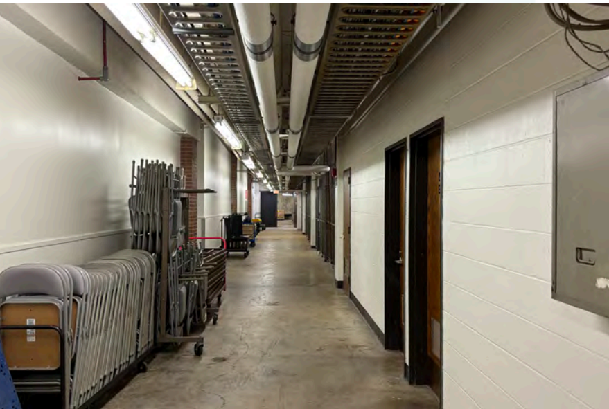
Utilities connect to most buildings via a series of underground tunnels, which allows for easy inspection and maintenance
