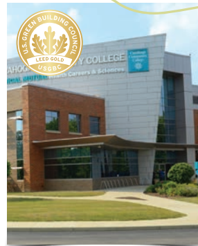
Westshore Campus Health Careers and Sciences LEED Gold, December 2012
