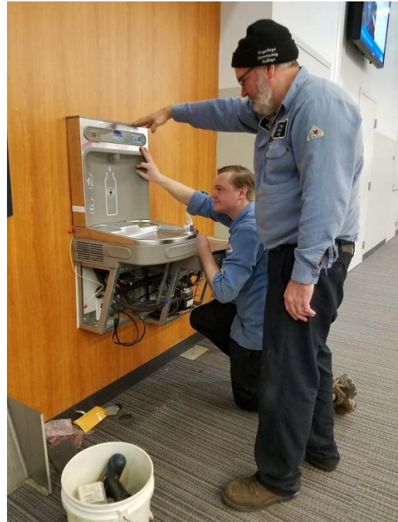
Employees install a water bottle filling station at the Eastern Campus
